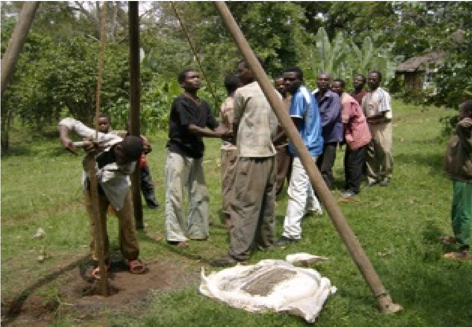
Project in Process
